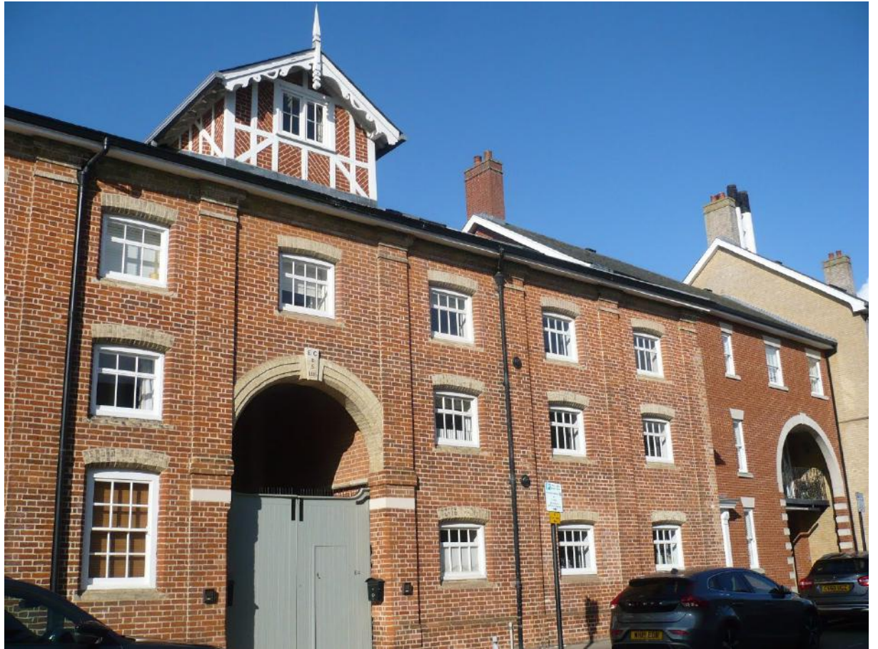
Image showing converted Maltings, College Street, Bury St Edmunds
