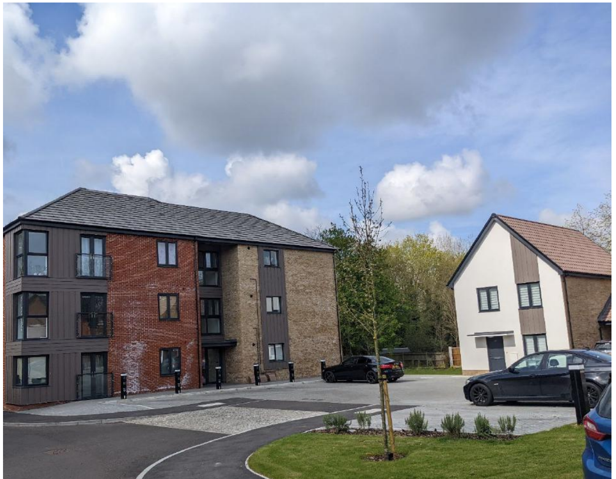
Image showing Barley Homes development Westmill Place, Haverhill
